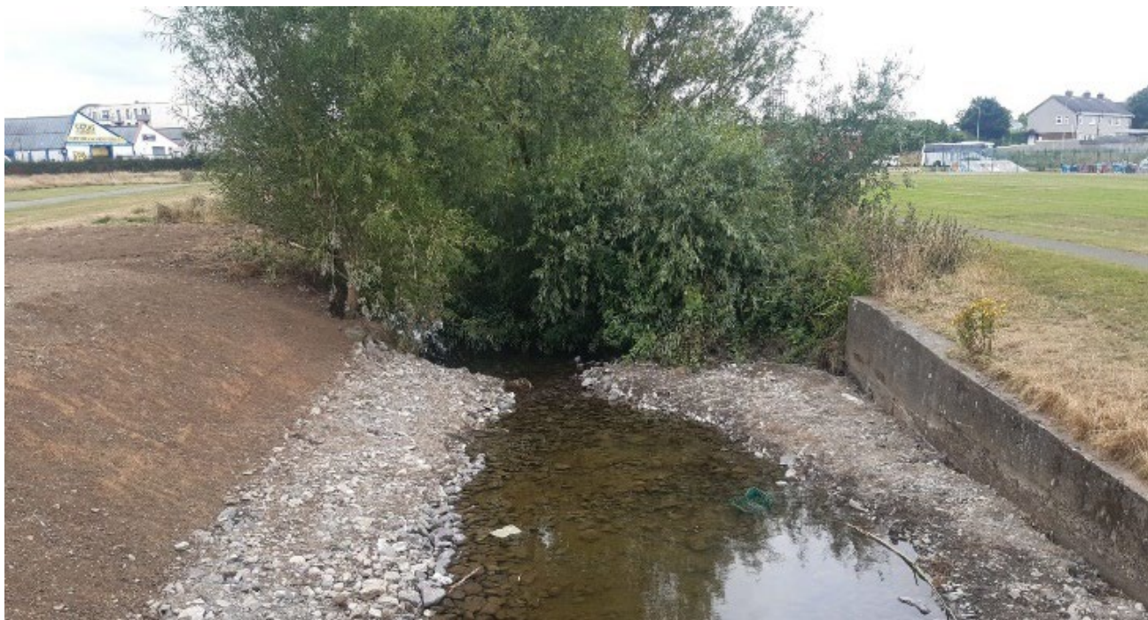
Weir Removal River Ward
