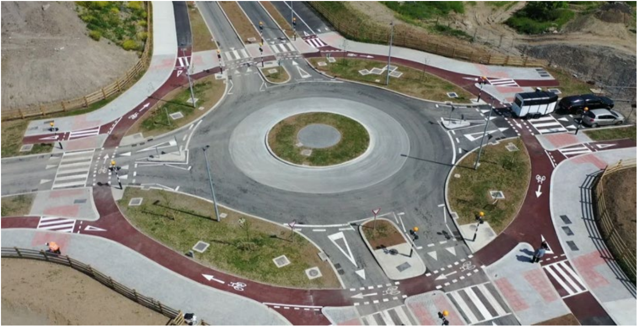
Churchfields Link Road with 'Dutch style' roundabout
