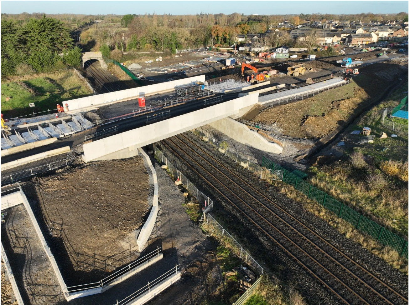
Ongar Barnhill Road Construction showing bridge over railway -December 2024.
