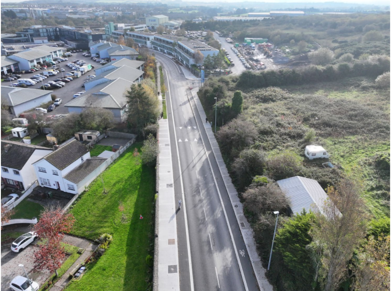
Harry Reynolds Road Pedestrian and Cycle Route - Substantially Complete – Jan 2025
