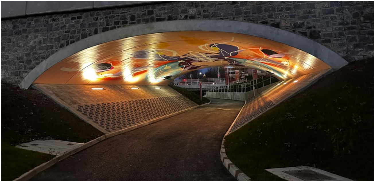
Snugborough Interchange Upgrade - Underpass.
