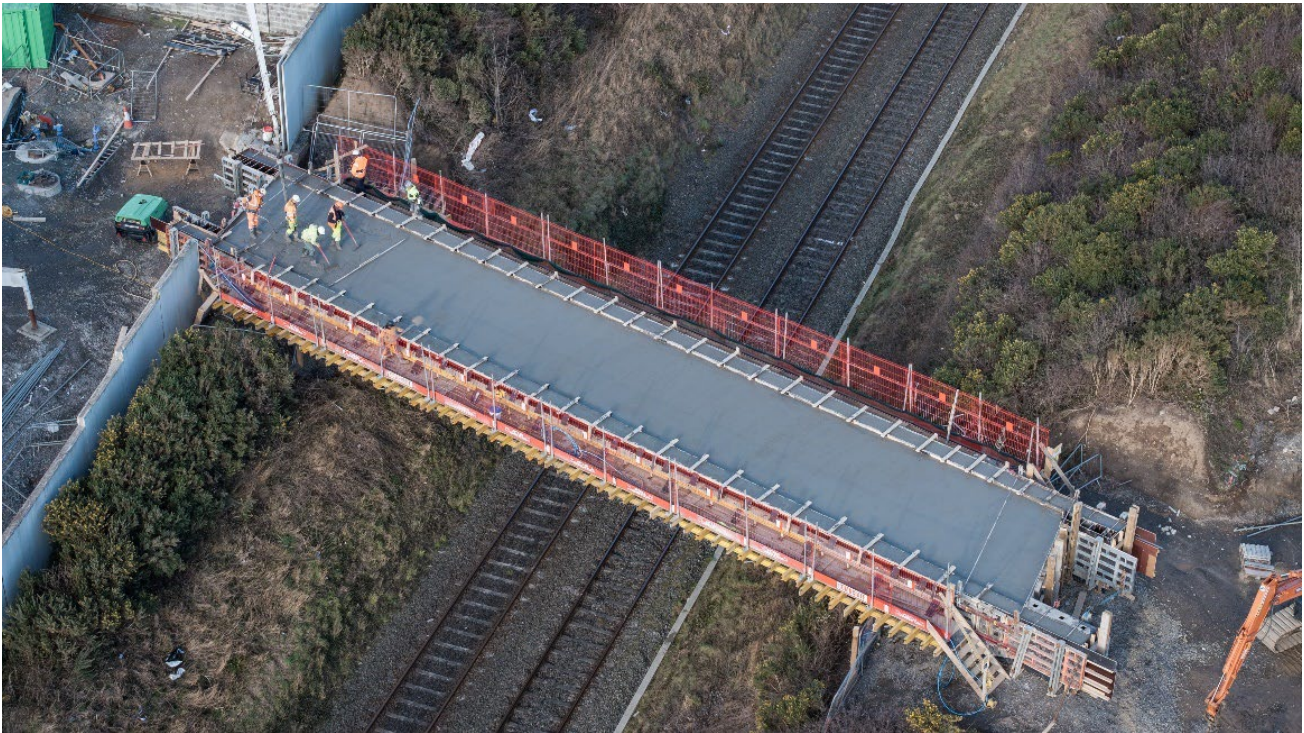
Donabate Pedestrian and Cycle Bridge under Construction
