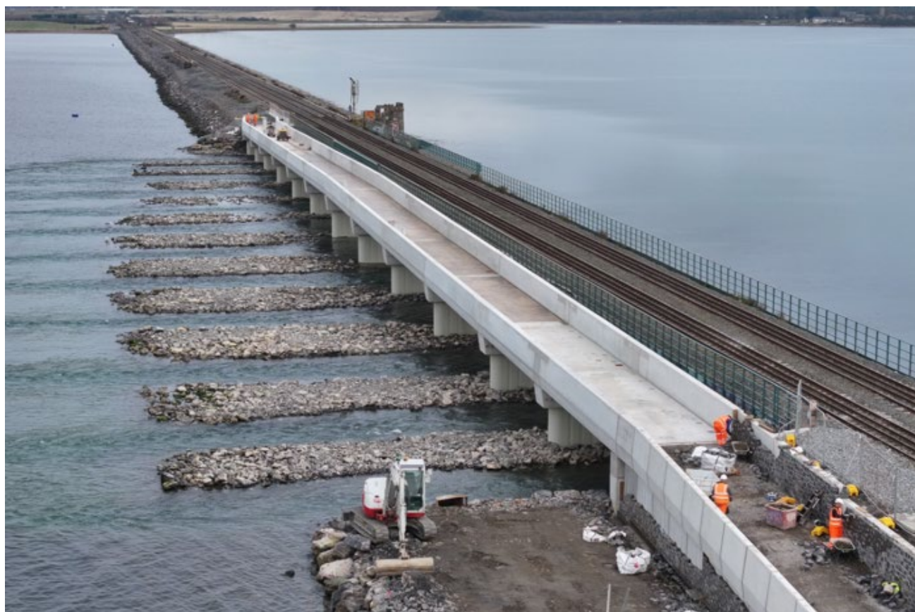
Broadmeadow Way Project showing the installation of the main estuary bridge.
